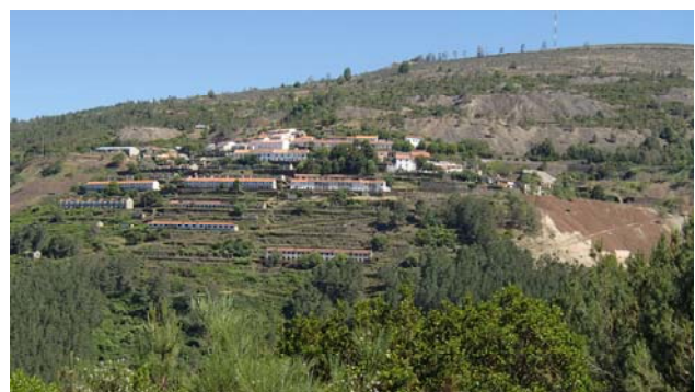
Fig 6. Waste piles over the old gallery entrances – Panasqueira Village.
