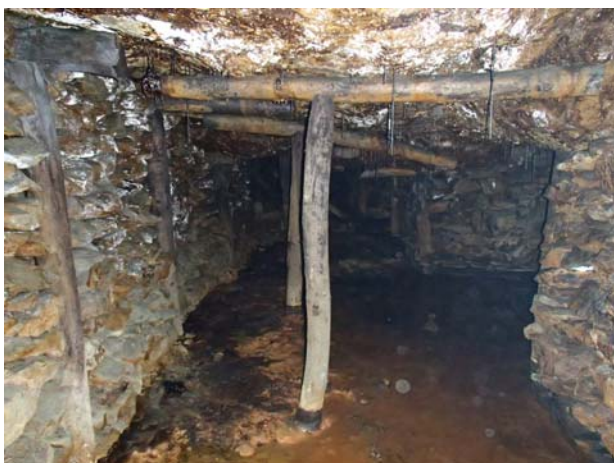
Fig 7. Old adit with rock wall made of waste.
